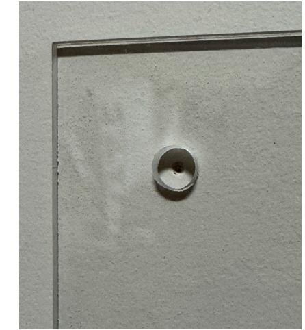
Use a 1/2" Center Punch to accurately transfer the center of each drilled hole to wall to locate wall anchors.
